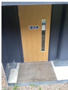
Front west fire exit
