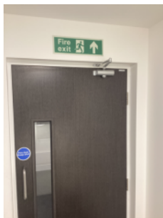
Fire exit sign in the lower ground lift lobby
