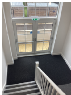
Fire exit door (to the east side of the building)
