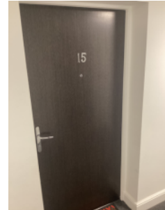
Flat 15 front entrance door
