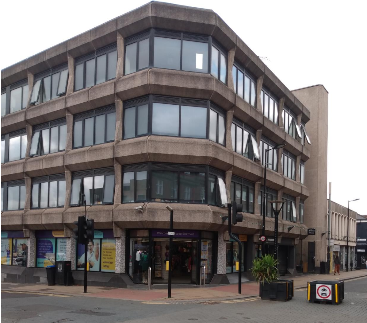
Division House, Sheffield
