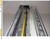
Breach in compartmentation where cables vertically pass through ceiling / floor. Potential for heat, smoke and/or fire to spread from the point of origin to further parts of the property.
